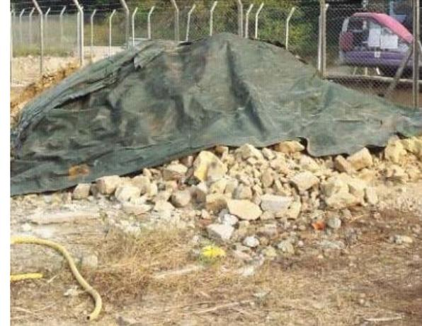
*Photo 4 - The corrective action to cover dusty materials was conducted by the Contractor in the following day of site inspection.*
